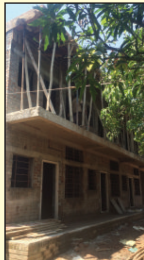
Roof Casting 1 st Floor
