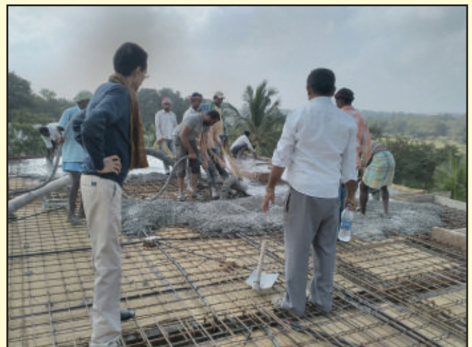
Roof Casting of 2 nd Floor
