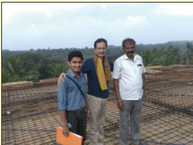
With Atheesh, Builder Rajanna on 2 nd Floor Roof - Dec. 15
